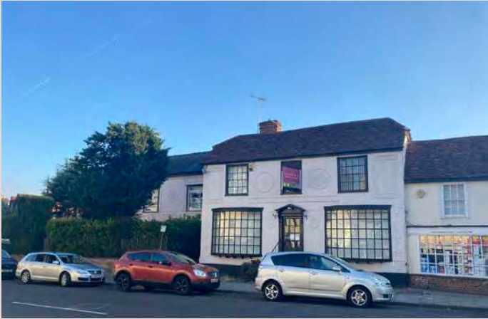
▲ Former shop retains pargetting and bay windows to enhance ornate character of new terrace home - High Street, Great Dunmow.
