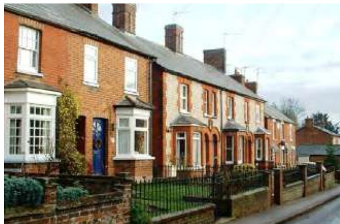
▲ The railway opening in the area meant a range of materials could be used for simple, yet-high quality house building in the 19th and 20th century. Picture above Bentfield End Causeway.
