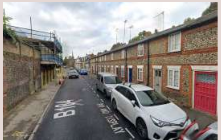
▲ Mirroring retaining stone walls materials creating a strong sense of character on B184.
