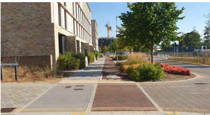
▲ Segregated cycleway, with landscape buffer to vehicular corridor and clear priority for pedestrians and cyclists at junctions.
