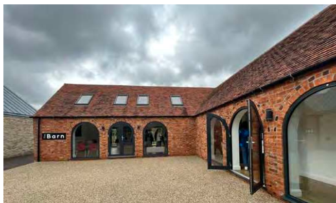
▲ New community facilities at Houlton, Rugby provided within former barn buildings.
