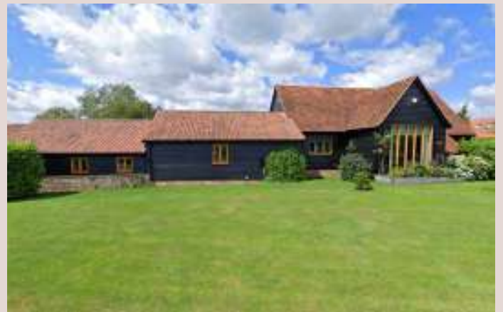
Local farmstead vernacular (black weatherboarding, peg tiled roof and flint wall) in Baconend Green.
