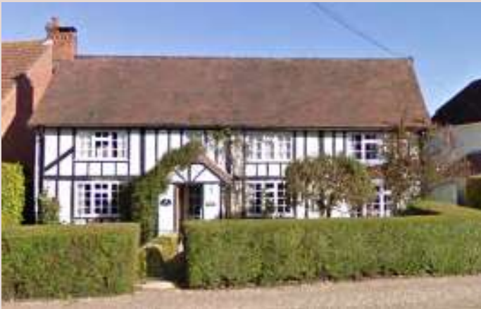
▲ Timber framed cottage with peg tiled roof overlooking Bannister Green. Low hedged boundary treatment integrated with informal shared space.
