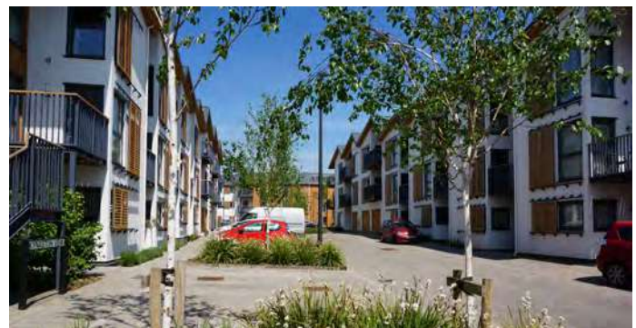
▲ Whilst continuous frontages are important they must ensure there is a minimal risk of overshadowing and a loss of privacy like here in Hanham Hall, Bristol.
