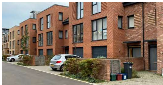
▲ Each dwelling in Reynard Mills, Hounslow has enough space for several bins as well as on-plot parking.
