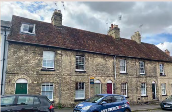
▲ Victorian terraces with peg tiled roofs and central chimney stacks on Gold Street.
