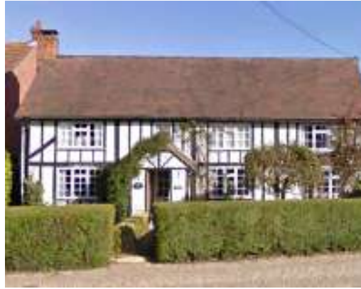
▲ Timber framed cottage in Bannister Green.
