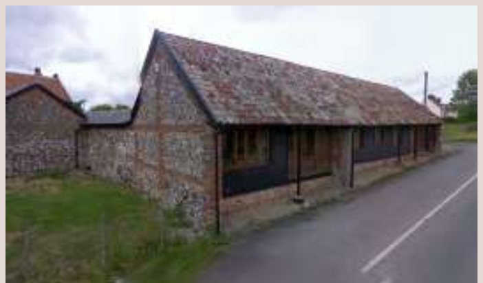
▲ Barn conversion using black weatherboarding with peg tiled roof and stone wall material at High Street, Chrishall.
