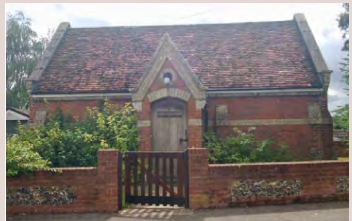
Little Chesterford village hall with red brick walls, front gabled entrance and clay peg tiled roof.
