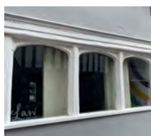
Wooden framed windows
