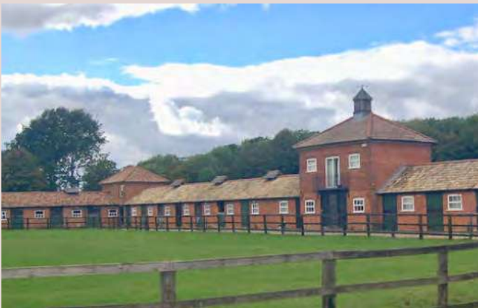
Individual single-storey stables at Brookend Farm Stables. Central two-storey block - built with red brick, projecting wings and gabled tile roof.
