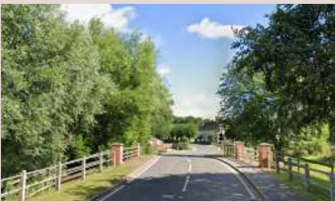
▲ Bridge over the River Pant lined with mature trees creates sense of arrival upon entering Great Sampford.
