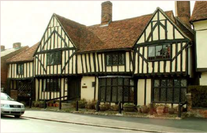
▲ Timber frames and peg tiled roof on Lower Street.
