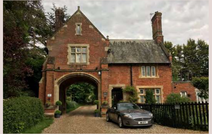
▲ Gatehouse with carriage-arch.
