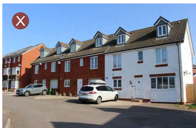
▲ Parking in front of dwelling with no trees or planting to reduce the visual impact.
