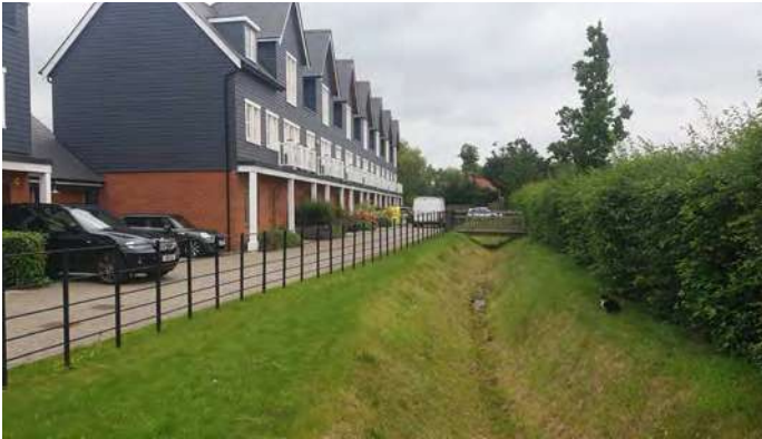
▲ Beaulieu, Chelmsford. Rural lanes integrate with swale features and existing hedgerows, similar to the protected lanes of Uttlesford.
