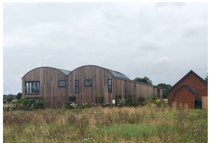
▲ Barn conversion in Uttlesford using prevalent vernacular materials.
