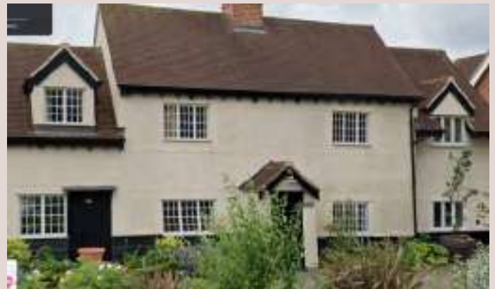
▲ Peg tiled roof, pargetting, dormer windows, central chimney and black weatherboarding Dunmow Road, Takeley.
