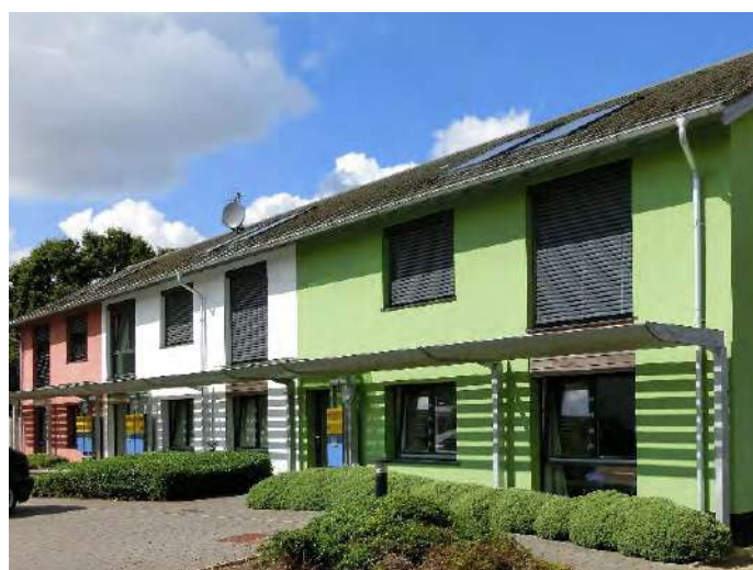
▲ Passivhaus development in Wimbish development by a local Housing Association where the properties are reserved for applicants with a strong local connection.
