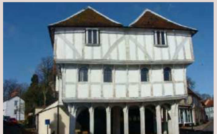
▲ Grade I listed Guildhall in Thaxted, ground floor forms open flagged market house with open timber ceiling, and heavy cross beams.
