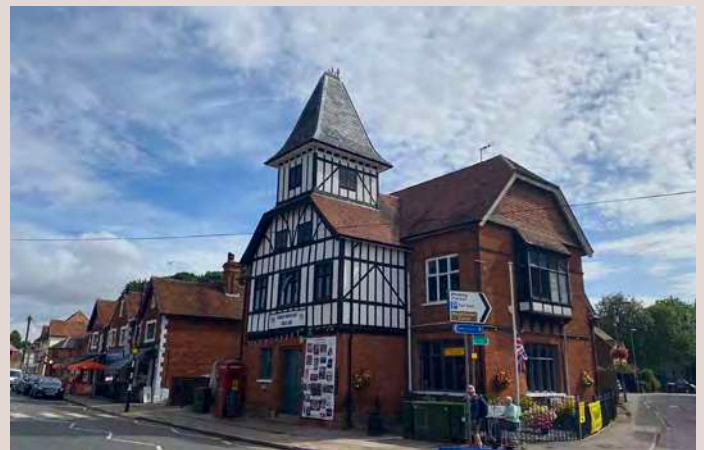
▲ Distinctive historic landmark aids wayfinding and acts as a gateway to the high street.
