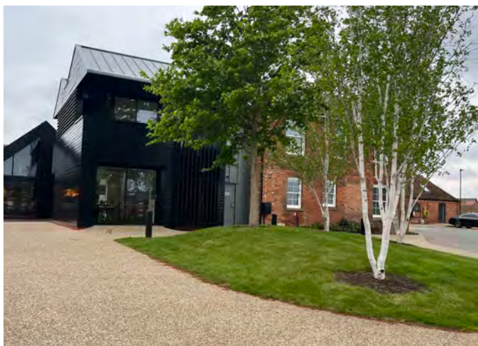
▲ Existing barn converted and extended to provide a visitor centre at Houlton, Rugby alongside community uses and a cafe.
