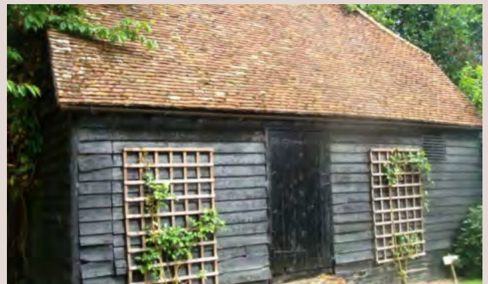
▲ Black weatherboarded barn with peg tiled roof demonstrates character at the smallest scale in Elmdon.
