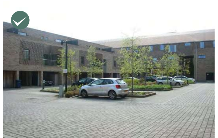
▲ Parking court with trees, planting and permeable paving.
