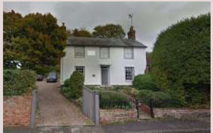
▲ Slate roof, white-washed plaster and simple iron railings - a common feature in Hadstock - on a half height flint wall in Linton Road.
