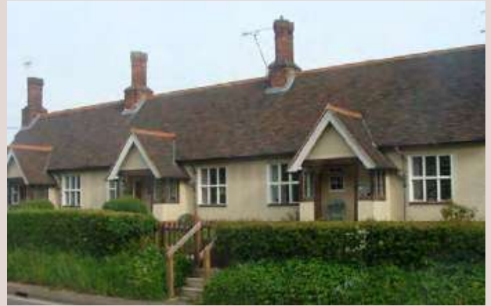
▲ Almshouses in Radwinter - Three gabled porches project on the front. Roofs tiled, with 4 chimney stacks each and casement windows.
