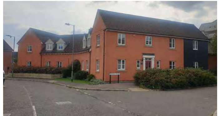
▲ Joined buildings at Flich Green create a compact development and make reference to local vernacular.
