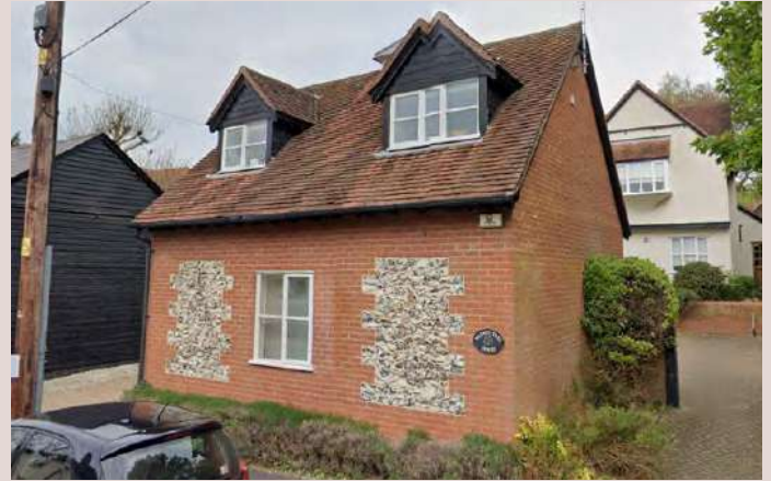
▲ Dormer windows and stone facade detailing on High Street, Great Chesterford.
