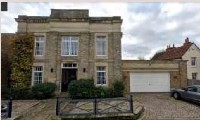
▲ The Chantry made from gault brick with pilaster features, is one of many church conversion examples in Uttlesford.
