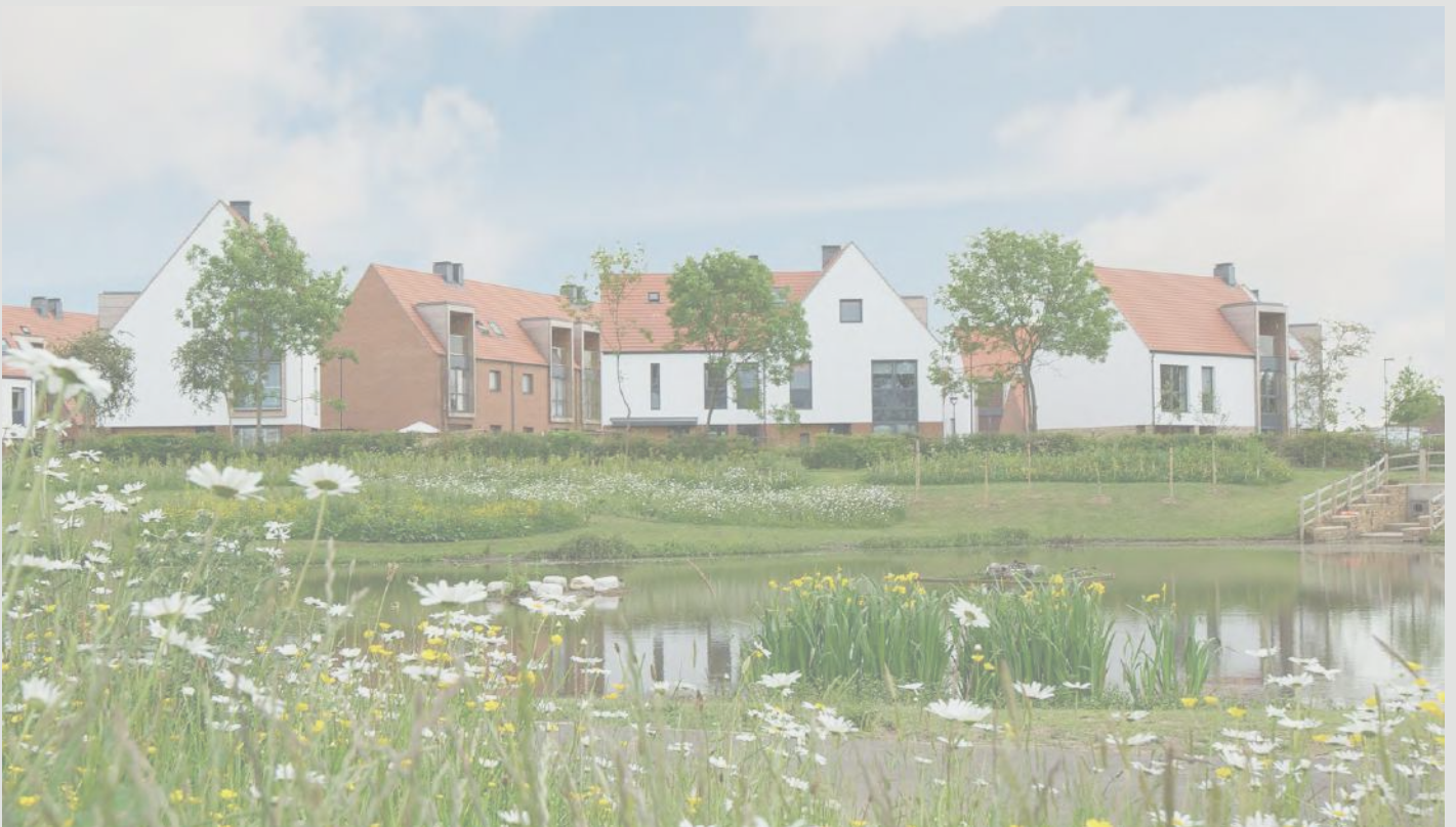
▲ Central pond provides a safe environment for breeding birds and wildlife whilst forming a key part of the sustainable drainage system and an attractive landscape feature, designed without a need for fenced edges
