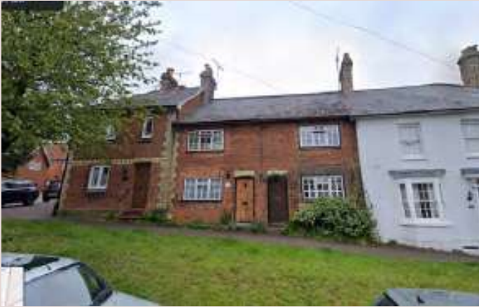
▲ Red brick terraces with barn doors opening onto Wicked Road, Newport.
