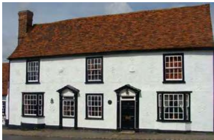
▲ The Bell in Great Easton, a former public house dating back to the 15th century, comprises of a timber framed building with pargetted facades.
